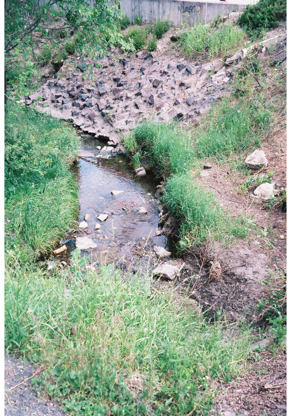
Figure 4 - Dry Gulch at Wadsworth Boulevard (east side)
