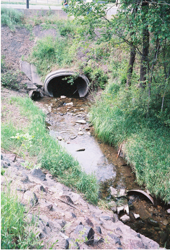
Figure 3 - Dry Gulch at Wadsworth Boulevard (east side)
